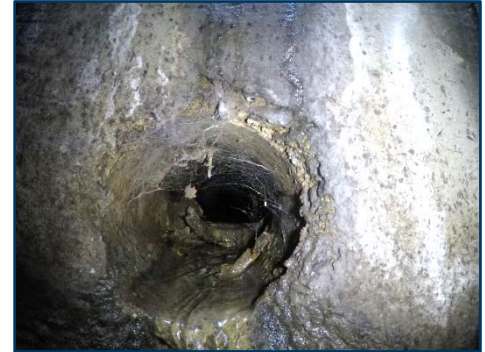
Collapsed Pipe
